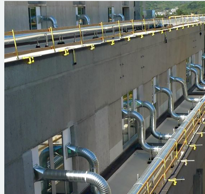
In response to COVID-19, many hospitals created temporary individual air handling units for patient rooms dedicated to COVID-19 patients. These rooms were converted to negative pressure to protect the staff and the rest of the patient population.
