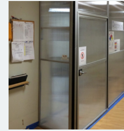
Portable anterooms can be added at entry to exam rooms for doffing space or to provide a negative pressure
