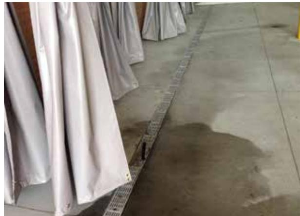
Fig. 3 b: Decontamination Shower Trench Drain
